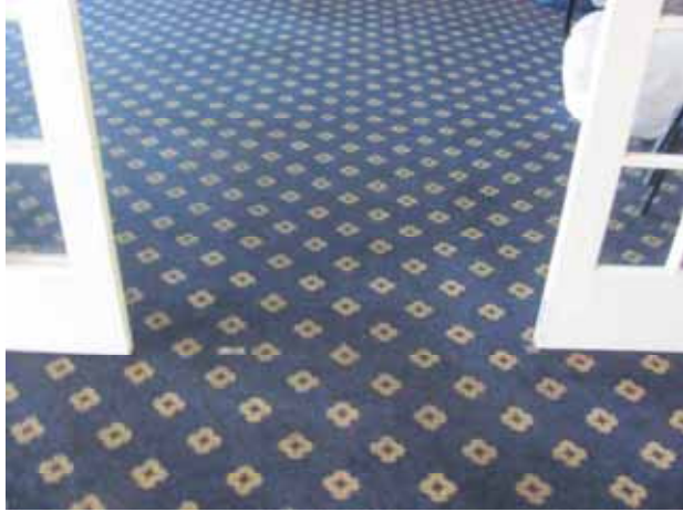
Carpet floor coverings at bay room
