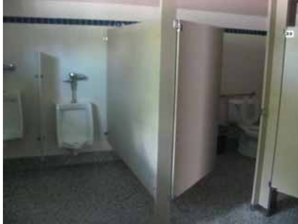
Pool cabana building
