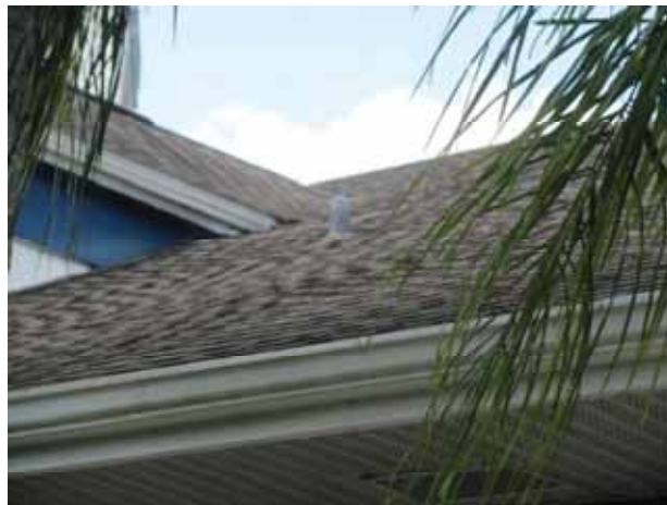
Asphalt shingle roof at clubhouse
