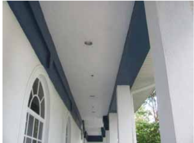
Painted stucco at clubhouse
