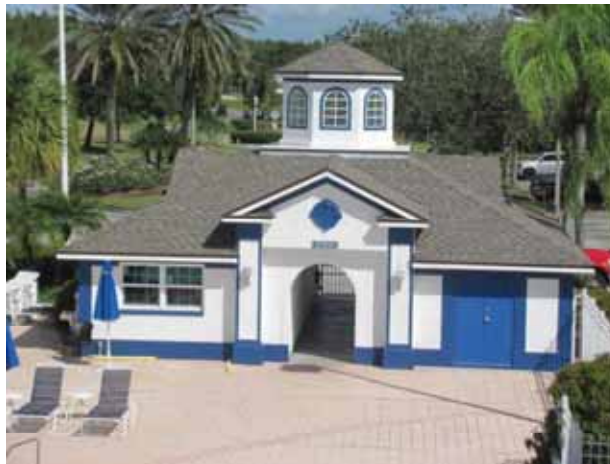
Painted stucco at pool rest room building
